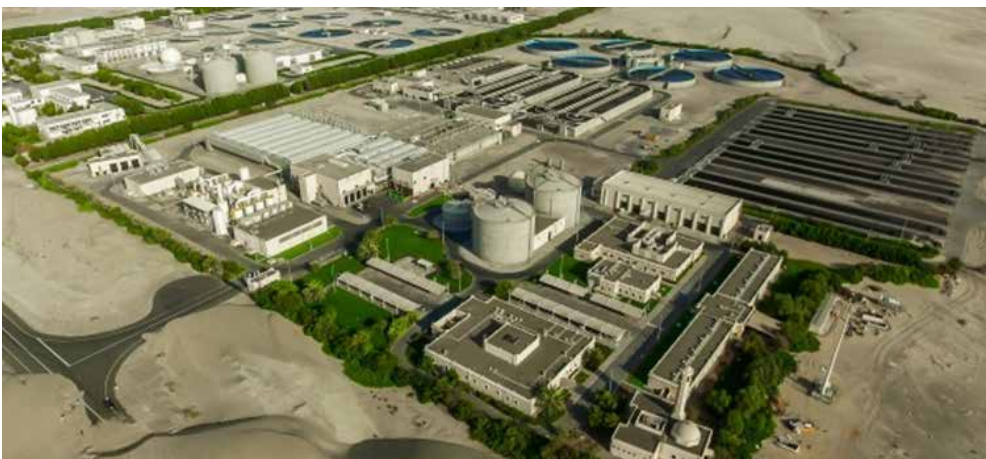
IMAGE 8.1 Al Wathbah-2 WWTP.
